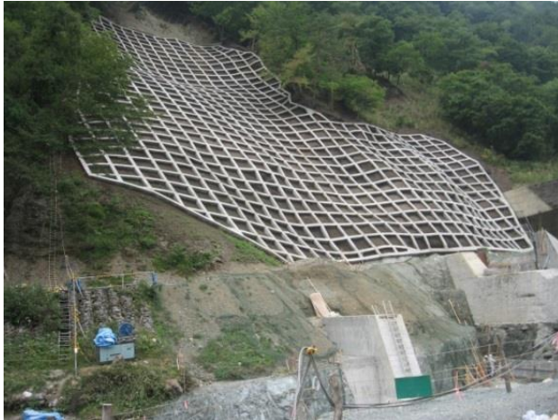
Figure 10 Landslide stabilization in Japan reduces the watershed sediment yield.
