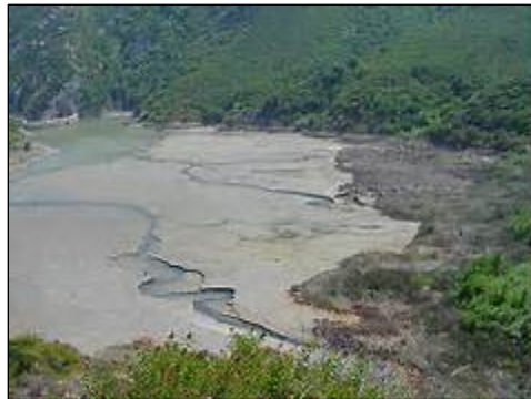
Figure 1 Sediment Deposition in Matilija Reservoir, CA (USBR 2010)
