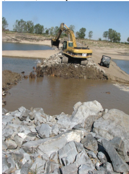
Figure 7, Dike Notching at Island 70
