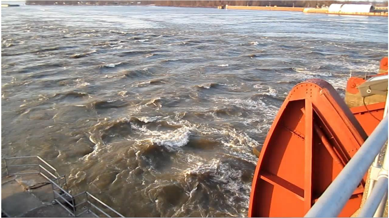
Figure 2 Downstream view of L&D25 on March 17, 2011 showing large standing waves
