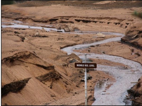
Figure 7 Loss of reservoir storage due to excess sediment deposition following the Waldo Canyon fire in the Monument Creek drainage.
