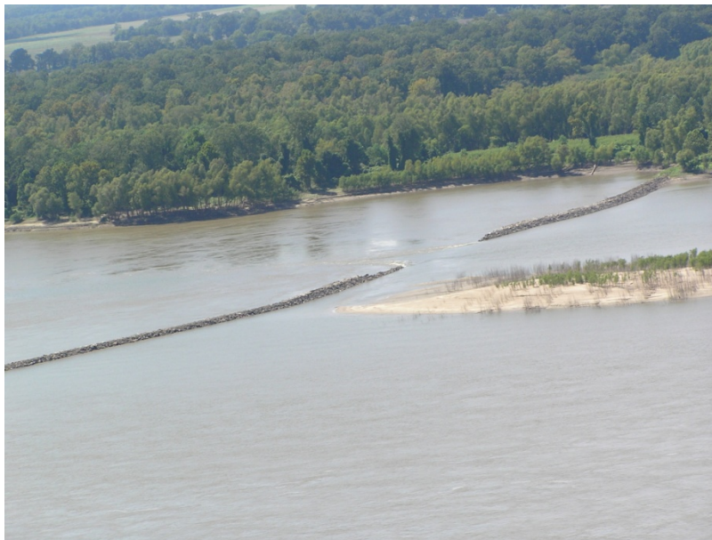
Figure 6. Mississippi River Notched Dike
