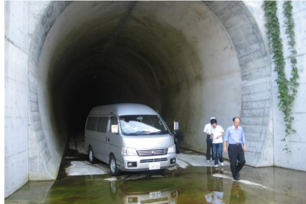
Figure 11 A tunnel was constructed along the Miwa Reservoir in Japan to bypass river flows with high sediment concentration.
