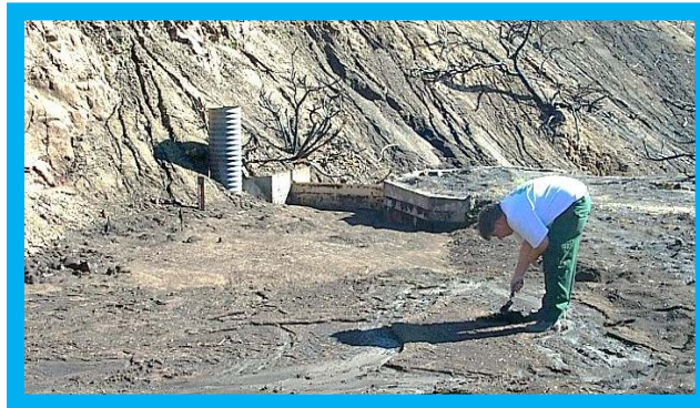
Figure 3 Debris basin for trapping small watershed sediment yield.
