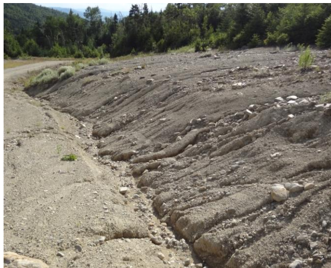
Figure 9 A recently constructed logging road on Elephant Peak, ME. The side ditch that was excavated into a till sheet illustrates an unvegetated, sloping surface that is undergoing gully and rill erosion. Photo by author.
