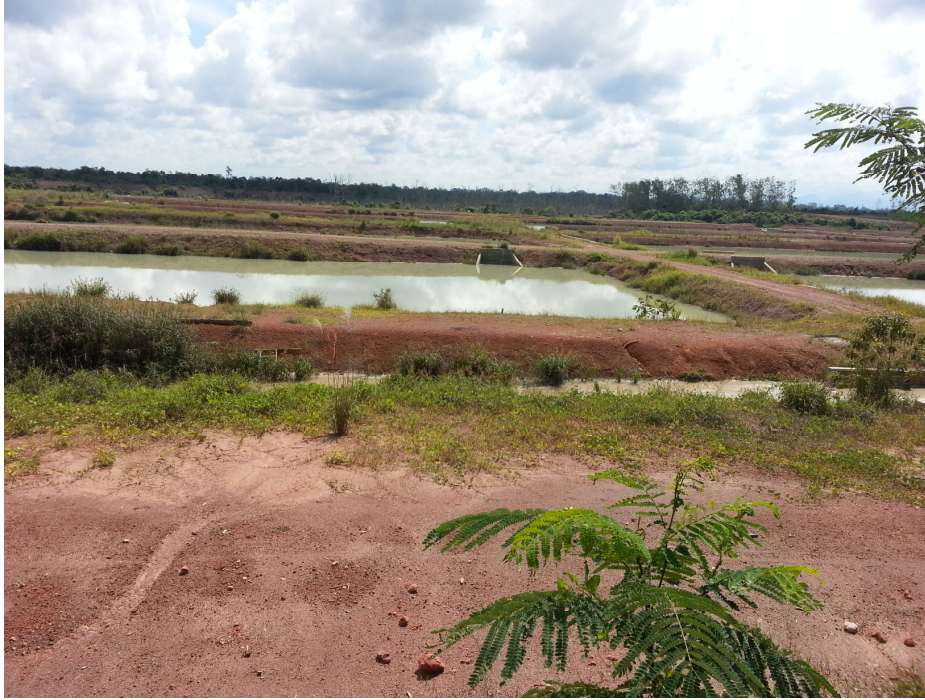
Figure 3 A series of sediment settling ponds surrounding one of the open-pit mines.
