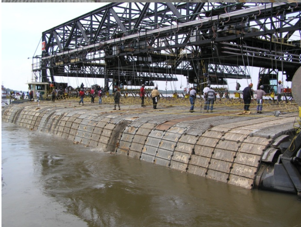
Figure 2. ACM Stacked on the Casting Field
