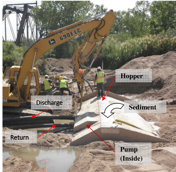
Figure 3 Sediment Collector™ at install.
