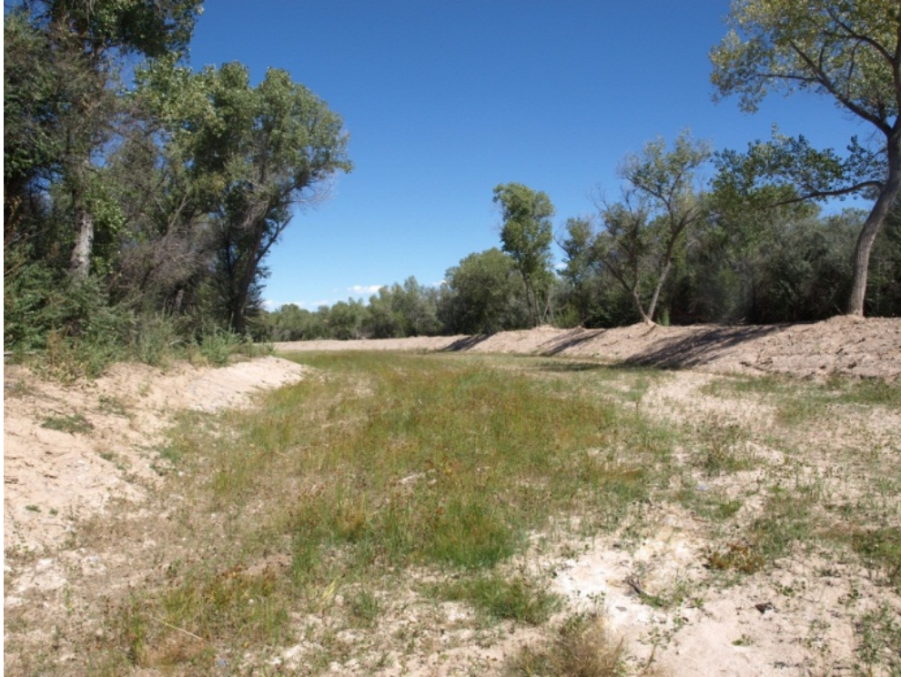
Figure 4 First season vegetation growth on bed of design channel near outlet of flow path 2, looking upstream. Photograph was taken on 10/1/2014.
