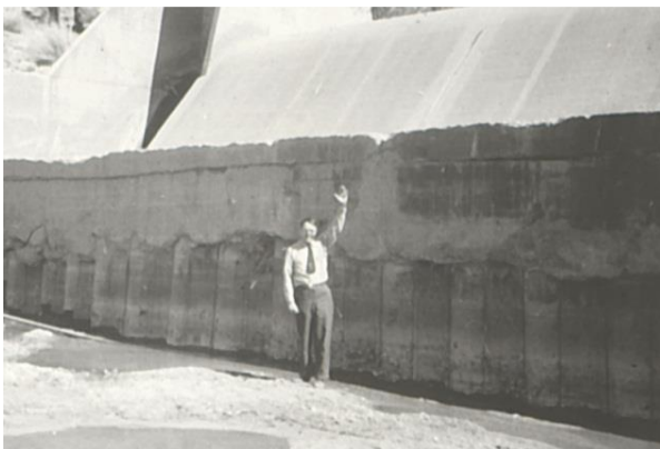
Figure 6 Channel degradation downstream from Sumner Dam near Fort Sumner, New Mexico.
