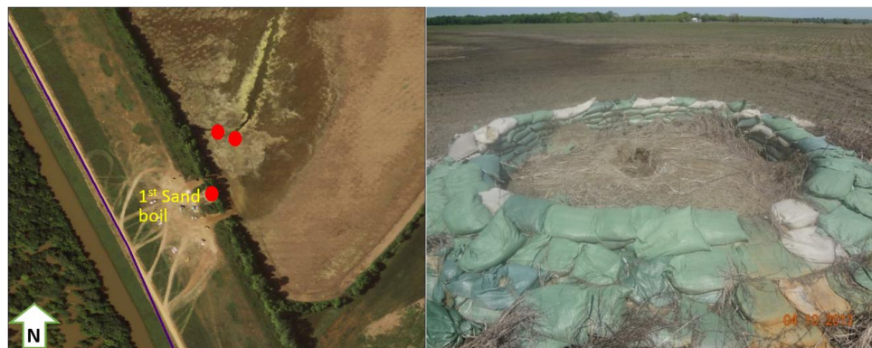
Figure 2 Location of sand boils (left) and mitigation of sand boil with sand bags (right)
