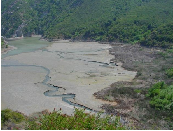
Figure 2 Sedimentation has almost completely filled the reservoir behind Matilija Dam near Ventura, California.
