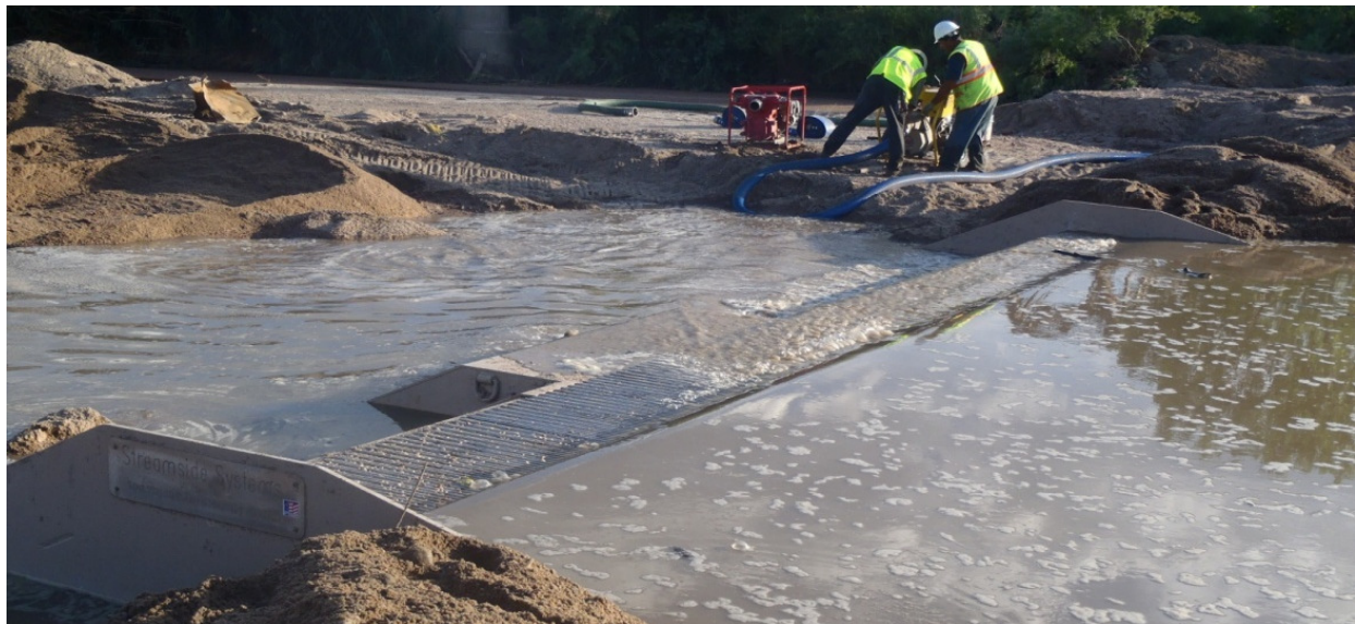
Figure 2 Sediment Collector™ installed in the dry in Fountain Creek.
