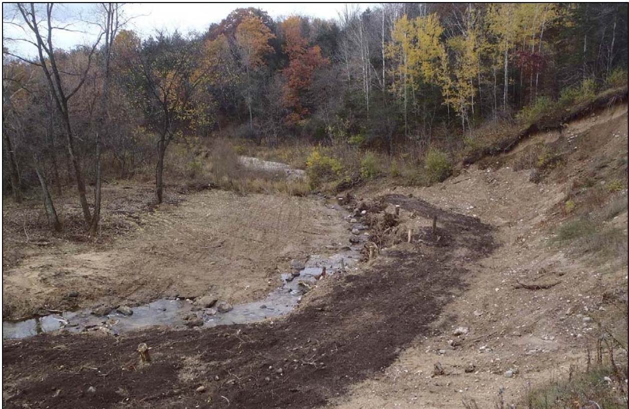
Figure 11 Photo of the Bluff 1 immediately after construction in October, 2013 (looking downstream).
