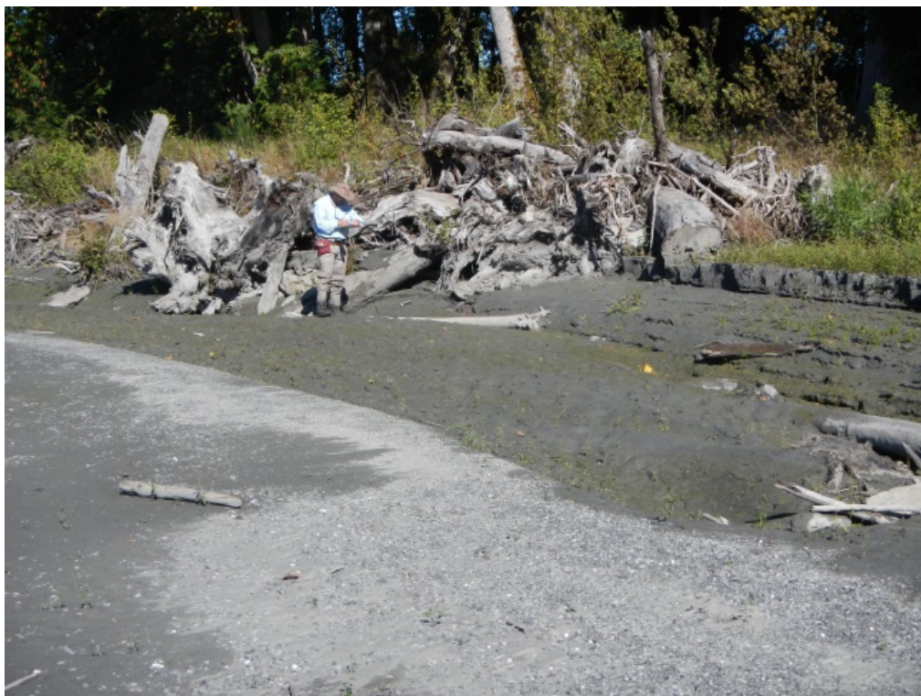
Figure 7 A new flat depositional surface is apparent around an ELJ.
