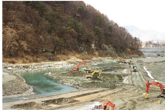
Figure 15. Mechanical dredging of reservoir sediments and transport by truck (Japan).
