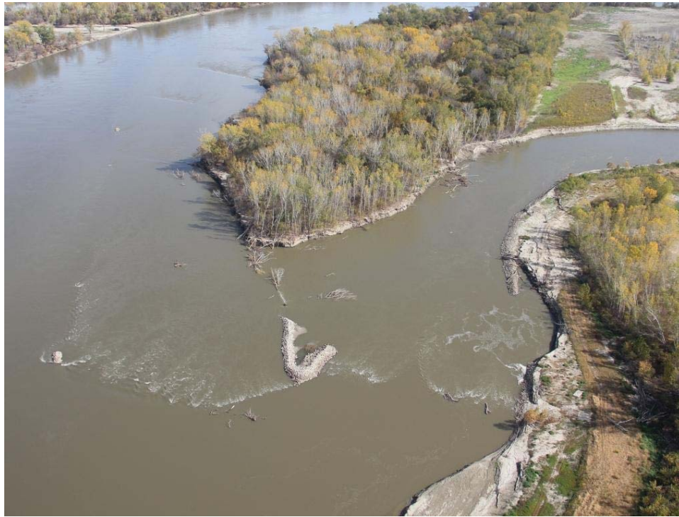
Figure 5 Typical Post Flood Chute Entrance Requiring Repair
