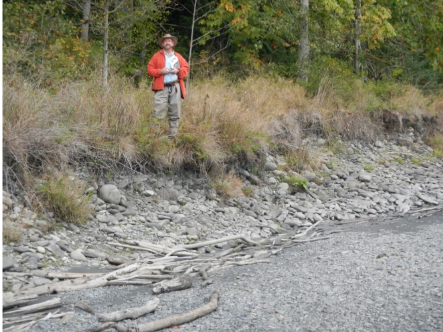
Figure 1 Downcutting shown in the left portion exposed an old channel, which is, now, a floodplain. The right portion of the image shows this old channels remnant floodplain as it was 50 years ago.
