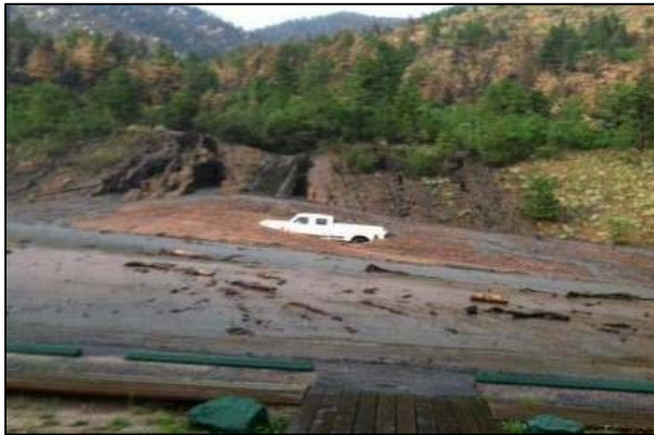
Figure 3 An alluvial fan being formed on Highway 24 following a post-fire flood. The flooding resulted in a fatality due to debris flows onto the highway.
