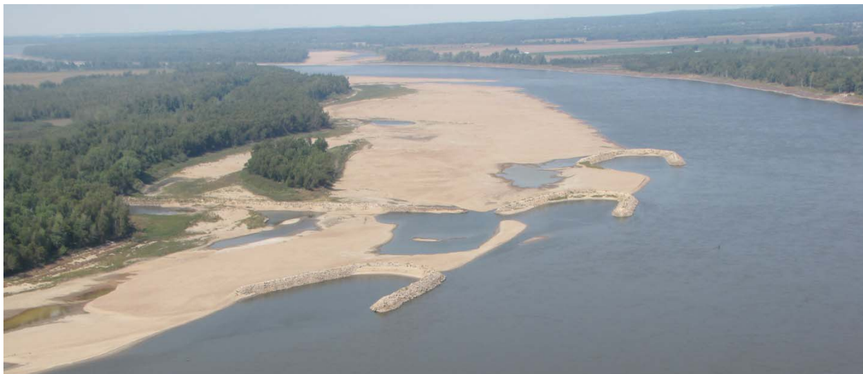
Figure 6. Chevron river training structures near River Mile 32.
