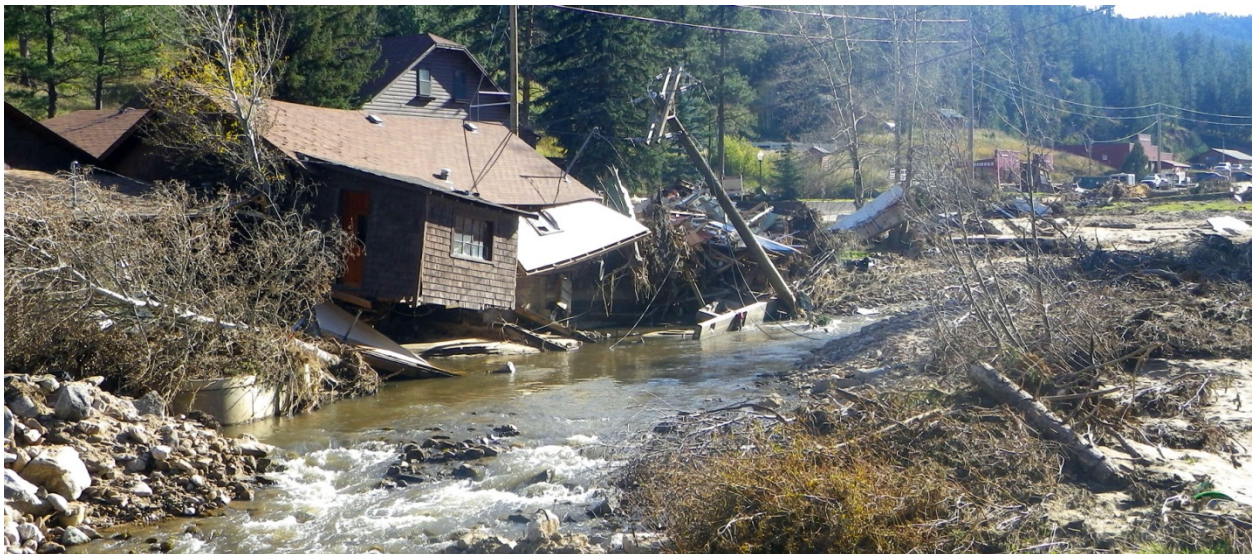
Figure 2 Flood damage in Glen Haven, along West Creek (photograph taken on 10/16/2013).
