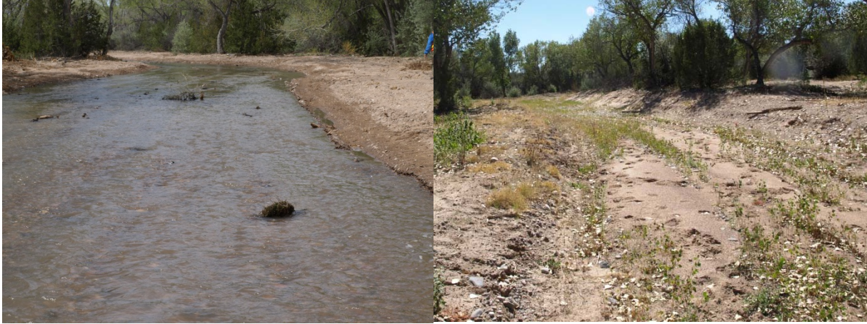
Figure 9 Looking downstream on one of the constructed channels. Left: Channel during spring runoff flows. Right: Channel after the spring runoff flows. Note the presence of sand deposits from upstream winnowing in the channel. Photographs were taken on 5/9/14 and 10/1/14, respectively.
