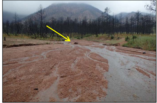
Figure 19 The debris basin completely filled with sediment and ash deposits, looking downstream on fan surface, North Douglas Creek (note the same exposed root wad and rock as shown in Figure 18).
