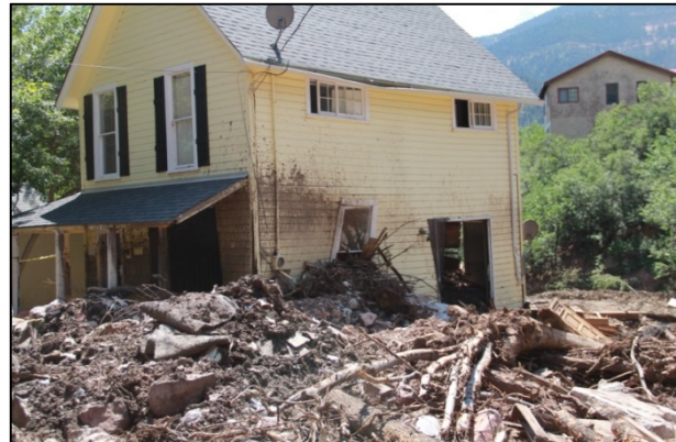
Figure 4 Destruction of homes following a post-fire flood and debris flow in Williams Gulch associated with the Waldo Canyon Fire.
